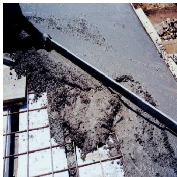
Pouring of Concrete
