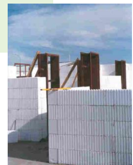
PLACING OF DOOR FRAMES
