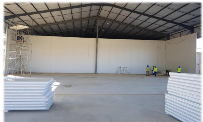
COLD STORAGE FACILITIES
